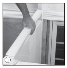
Place H channel over well wall (long ears). This channel should fit between wall plate and corner connector.
