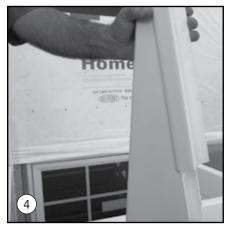
Slide H channel into side panel (short ears). Insert side panel into back plate. The nose should be flush with the front outside wall of the well.
