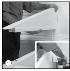
Secure panel to wall plate with 6 #10  $\times$  3/4" white screws. Secure panel to well with 6 #8  $\times$  1" white screws through long ears of H channel and 6 #8  $\times$  1" white screws through short ears of H channel.
