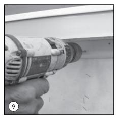
A header block is provided in the side frame box. Install on the bottom center, tight up against the header (to provide header support in the center).
