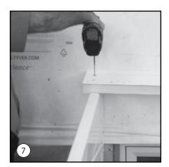
With side panels mounted, center header allowing approximately 3/4" overhang on each side, and secure with 2 3" SS screws at each end. Use the white plugs to conceal the holes.
