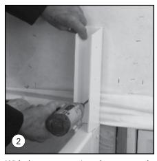
With the rear mounting plate centered over the well side and flush to the outside building wall secure with 2 Tapcons (3/16 x 1-3/4) while ensuring that the plate remains plumb.
