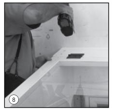
Brace the glass cap up to the header with the hinges facing up at the top. With the glass cap flush with the header edge, screw the hinge plate to the header with the black 1-1/2" screws.
