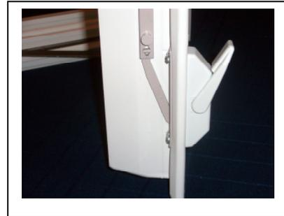
8. Loosen one and remove one screw from each of the two plastic strike plates on the locking side of the fixed main window frame.
